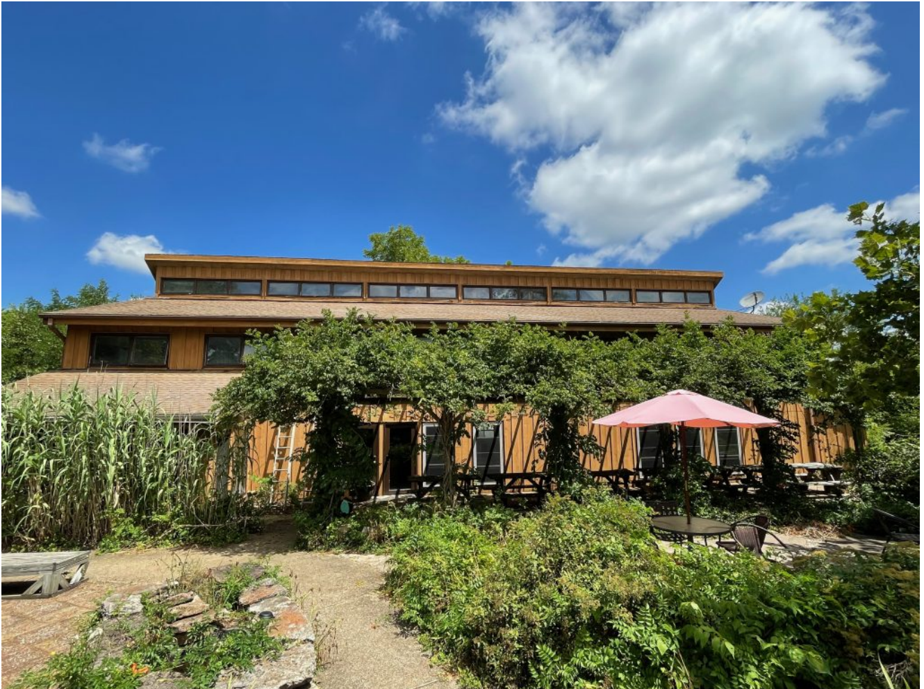
The Dining Hall roof
